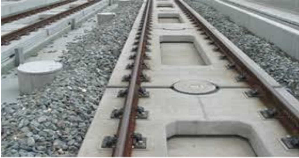
Figure 8: frame-shaped Shinkansen slab track system
