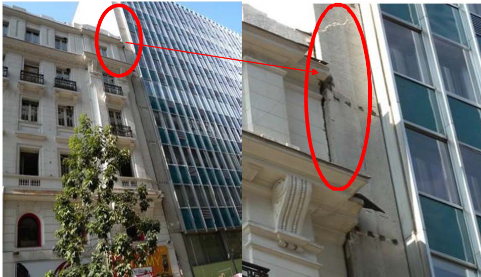
Fig 2.1: Pounding damage in Santiago due to 2010 Chile earthquake (photo by S.Brzez)
