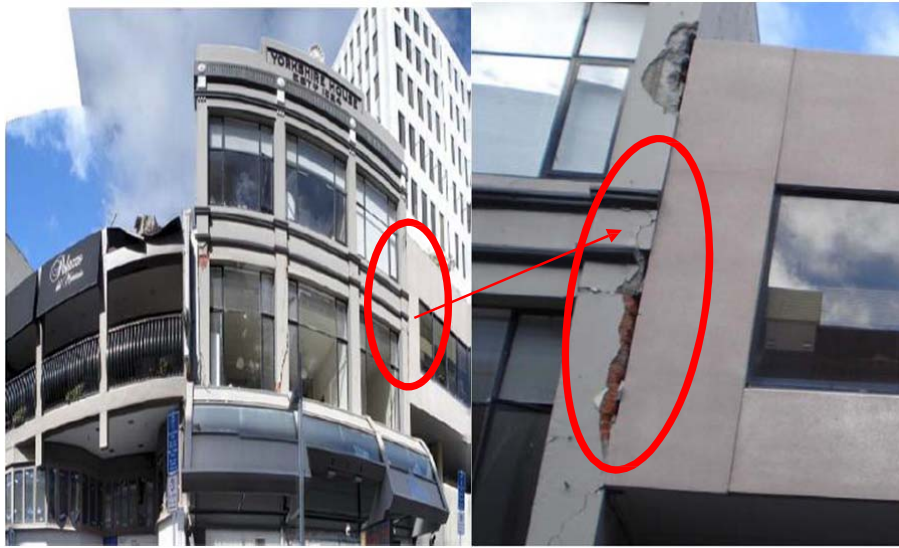
Fig 2.2: Pounding damage caused by different heights (photo by Gregory Cole)
