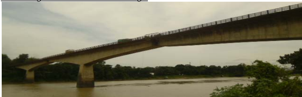
Other bridge in Silchar with central hinge.
